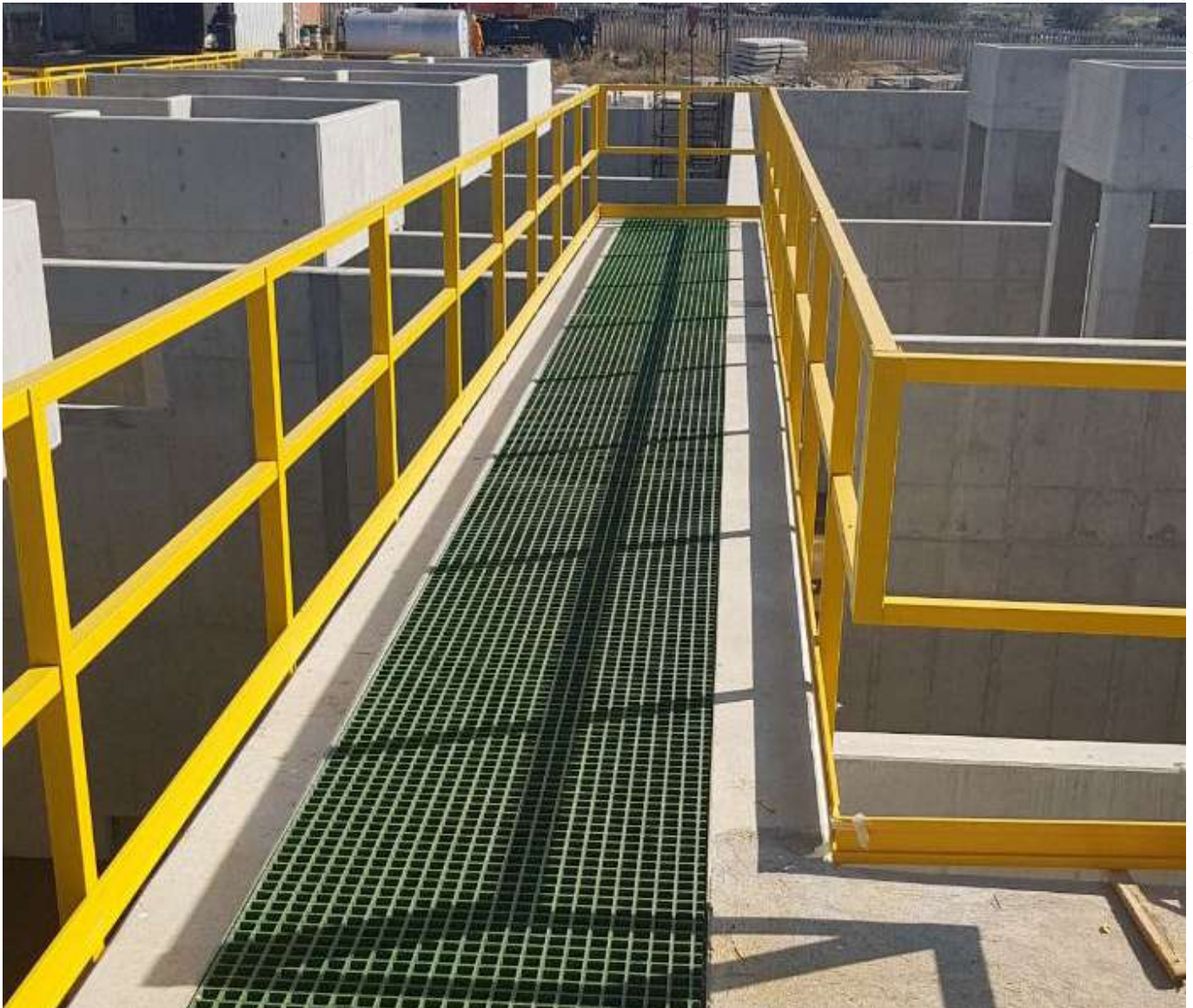
38mm GRP Grating and 44mm Square Tube Hand Railing
